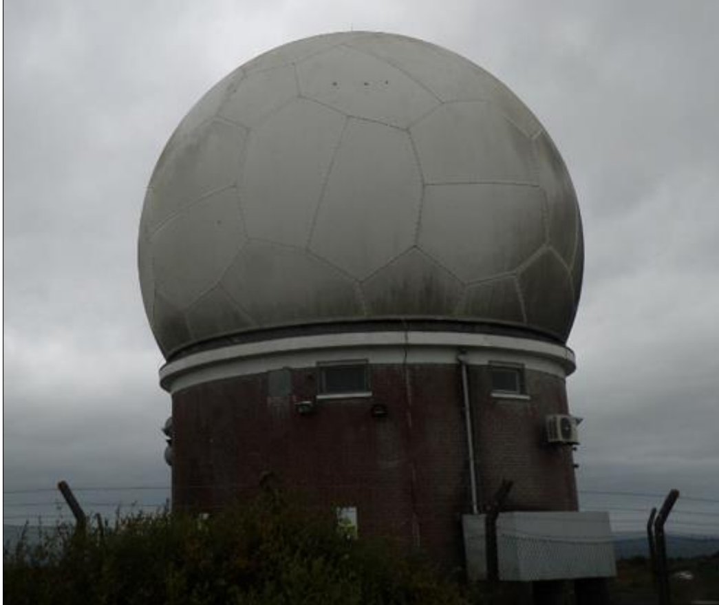
Figure 8. Woodcock Hill Radar Station
